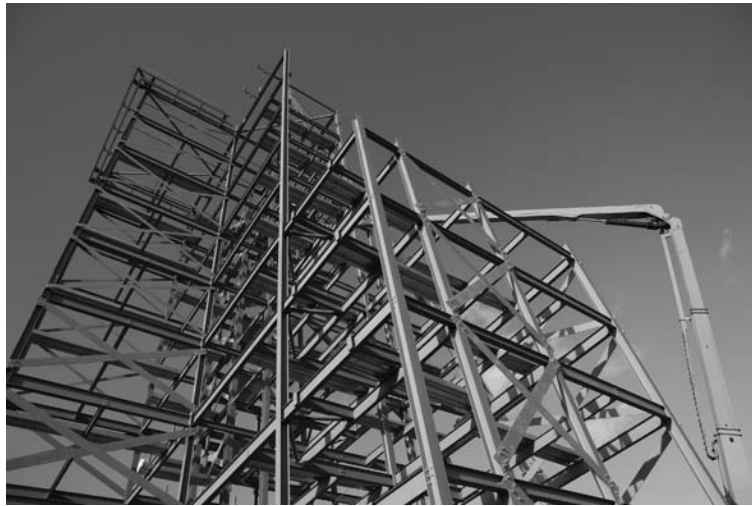
Fig. 1.4 Skeleton of a Structural Steel Frame Building
