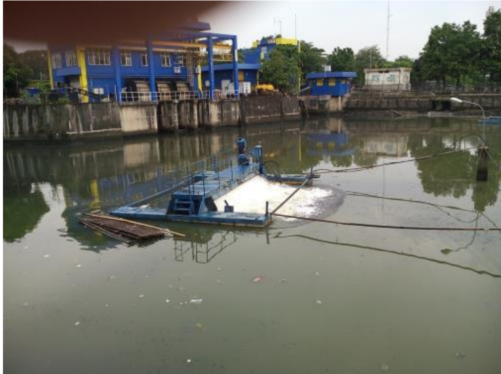
Gambar 3.5 Aerator ( Brush Aerator Surface )
