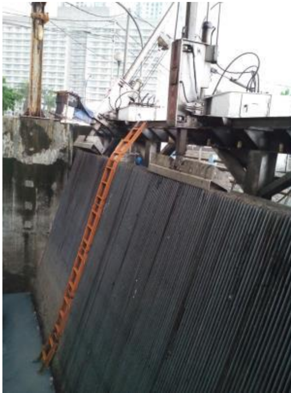
Gambar 3.4 Sistem Penyaring Sampah Otomatis ( Mechanical Bar Screen )
